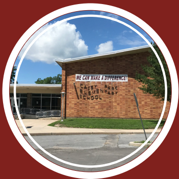
Casey Park Elementary School
