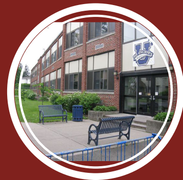
Genesee Elementary School
